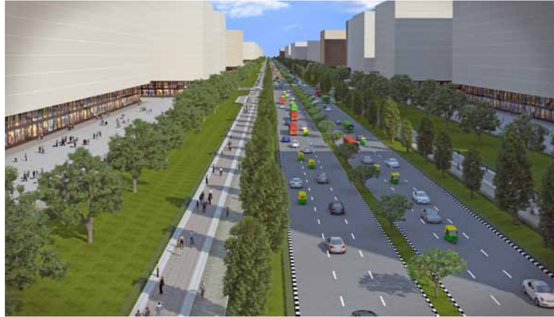
View of 40 m wide the existing Nangloi–Najafgarh Road that has been re-proportioned to accommodate all modes of transport with equal priority. The green verge along the road creates a buffer between the built edge and the road and allows for pedestrian friendly plazas and social spaces
